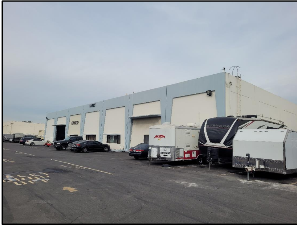
Plate 3.2-3: Overview of the industrial warehouse buildings from the southeast corner, facing northwest.
