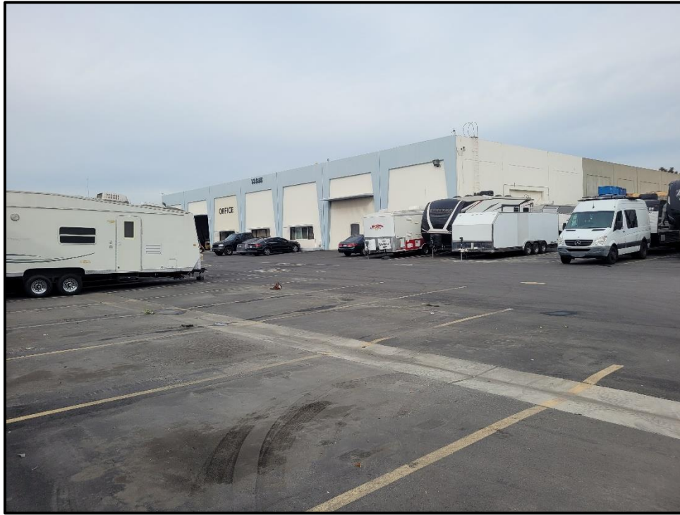
Plate 3.2-1: Overview of the project from the southeast corner, facing northwest.
