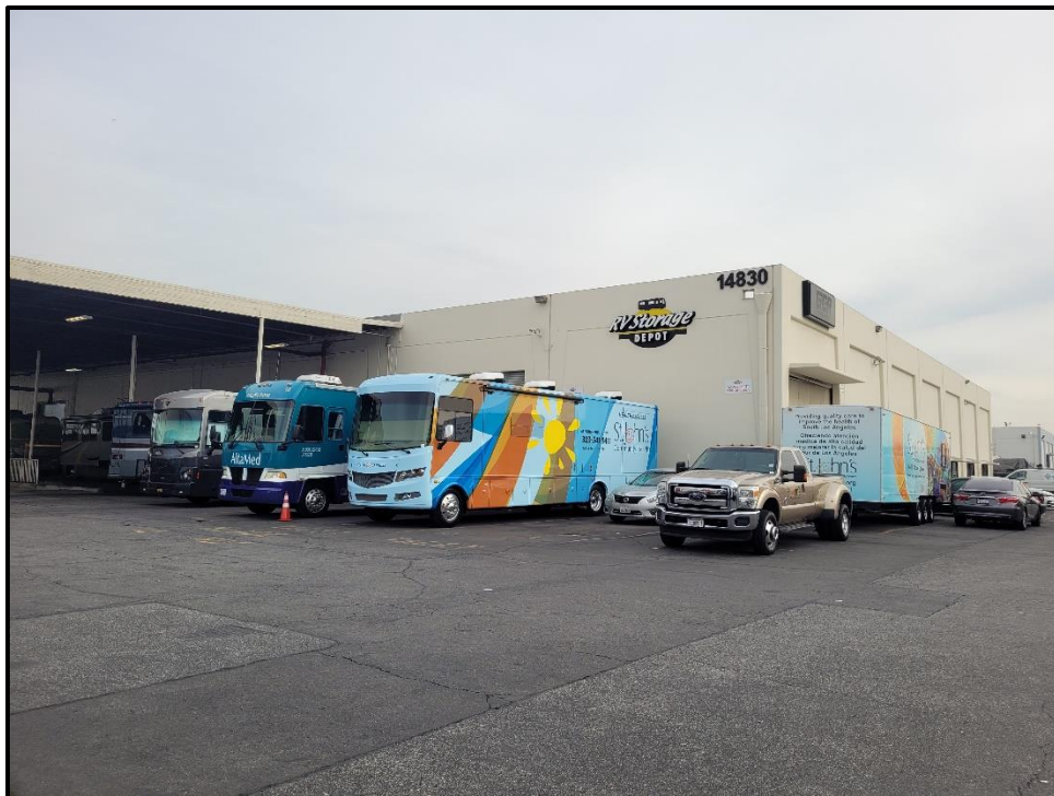
Plate 3.2-4: Overview of the industrial warehouse buildings from the southwest corner, facing northeast.
