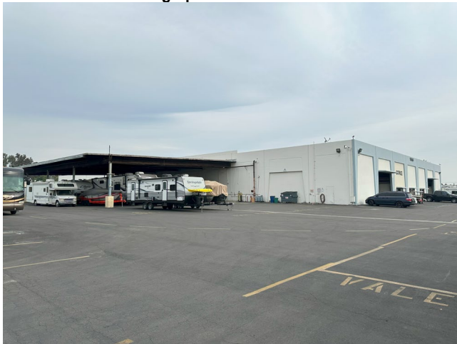
Easterly Bldg façade and W elevation canopy, view NE
