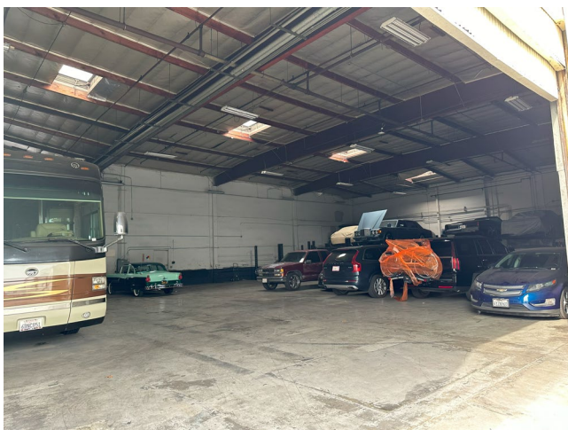
Westerly Bldg interior, showing skylights, view NW
