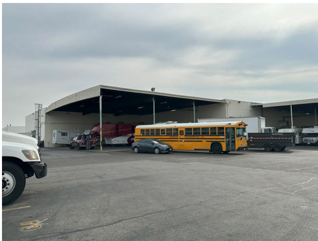
Westerly Bldg W and N (rear) elevations and canopies, view SE
