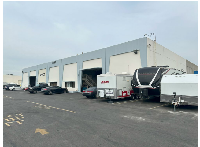
Easterly Bldg façade and E elevation canopy, view NW
