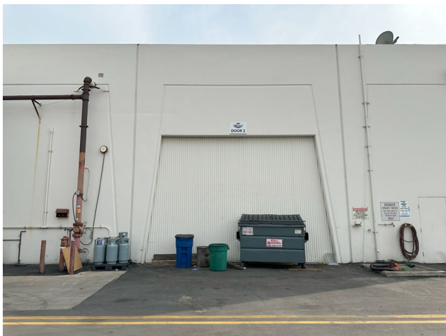
Easterly Bldg W elevation scoring detail, view E
