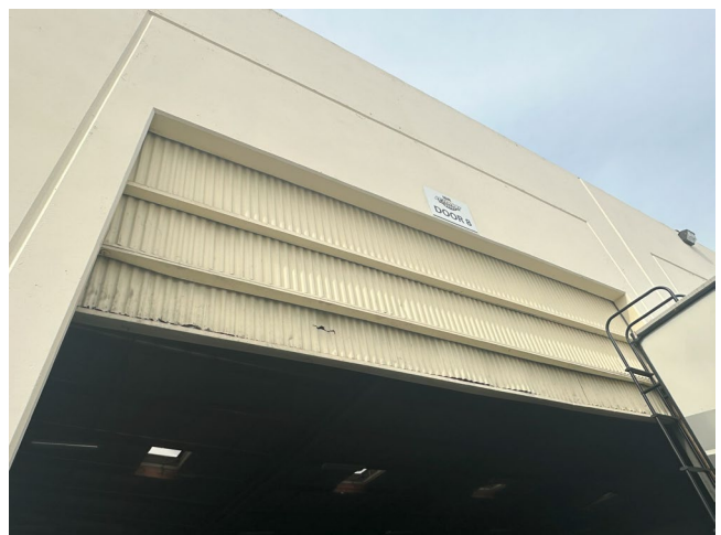
Westerly Bldg original telescoping door, view NW
