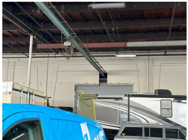
Westerly Bldg alteration detail, view E
