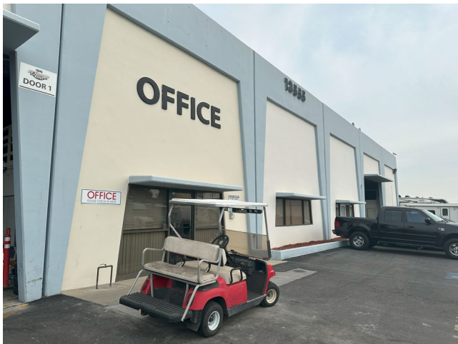
Easterly Bldg façade entry & fenestration, view NE
