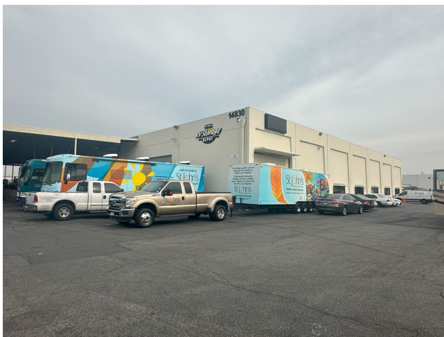
Westerly Bldg façade and W elevation, view NE
