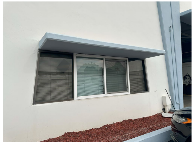
Easterly Bldg window, modified, view N/NE
