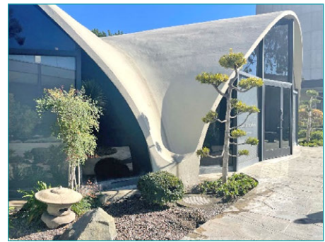
Figure 2-15: City Hall Courtyard
