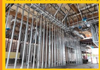
foundation work, structural steel installation, concrete masonry, and roofing. The interior is taking shape with metal stud framing.
