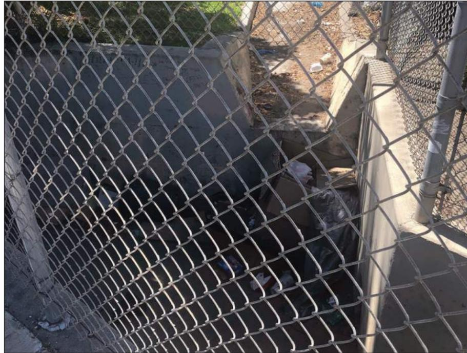
PHOTOGRAPH 10: Photograph of existing concrete-lined drainage channel with minor staining apparent.
