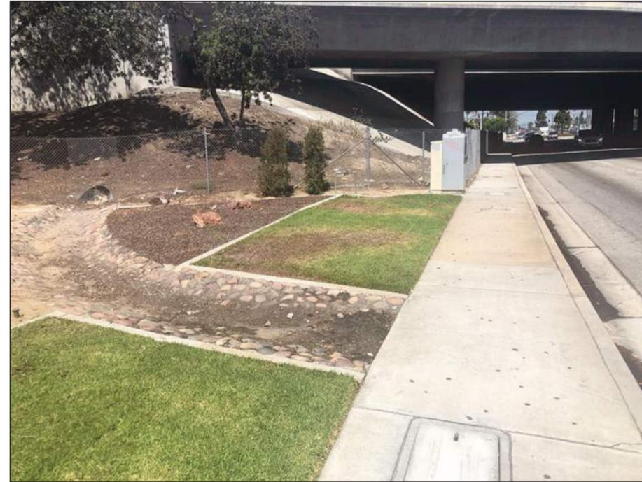
PHOTOGRAPH 6 Photograph of the existing stone-lined drainage ditch west and adjacent to the I-605/Firestone Boulevard interchange.
