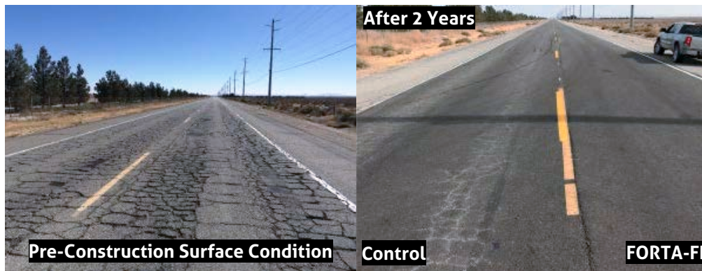
Figure 2. Reflective crack mitigation with FORTA-FI.
