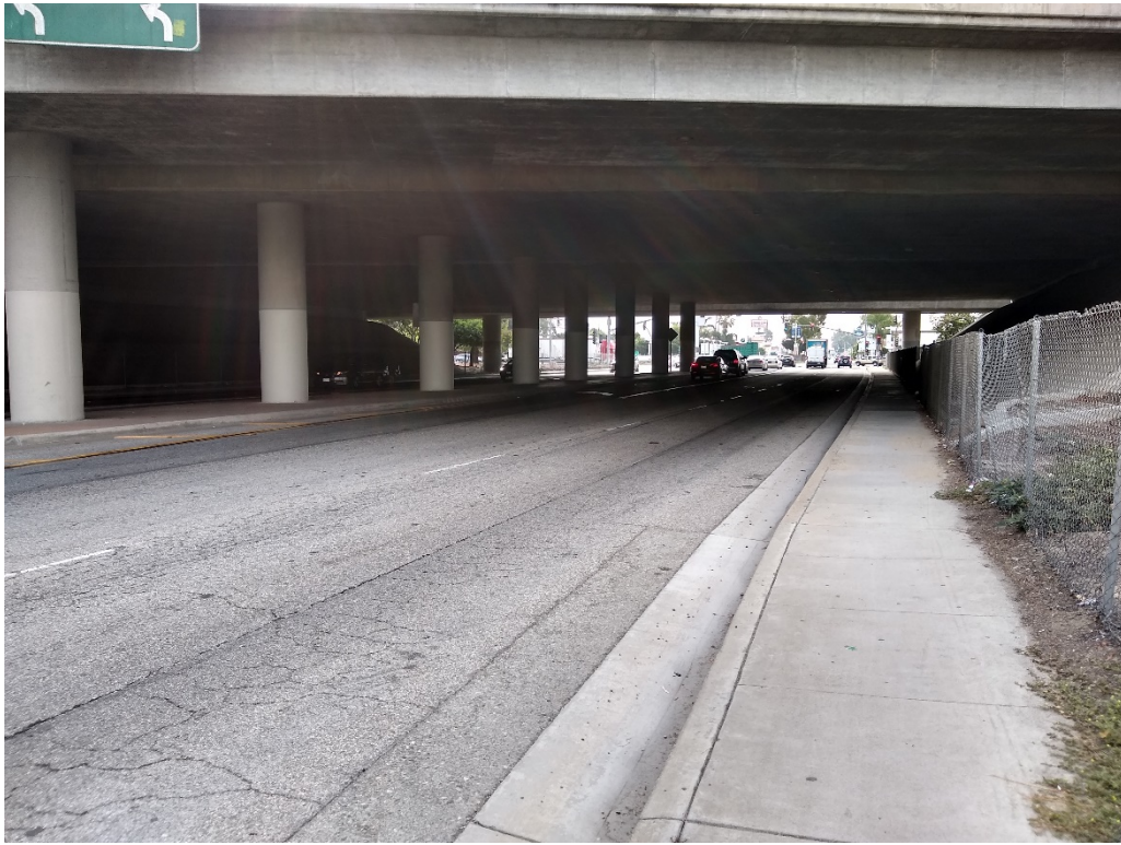
Photograph 1 – Firestone Boulevard under the I-605 bridge, facing northwest.
