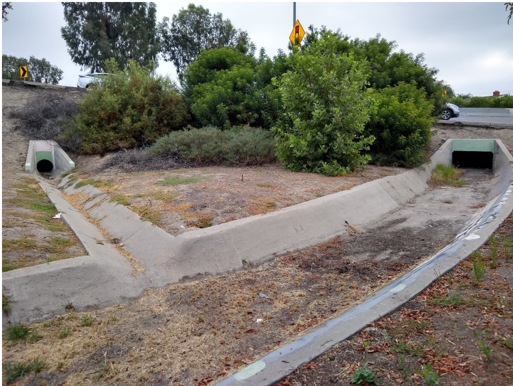
Photograph 8 – Concrete-lined drainage near the Firestone Boulevard I-605 northbound exit, facing north.
