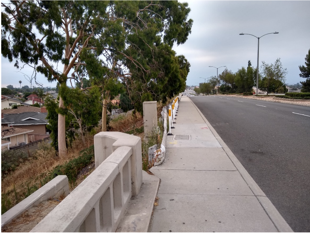
Photograph 5 – Firestone Boulevard, facing southeast.
