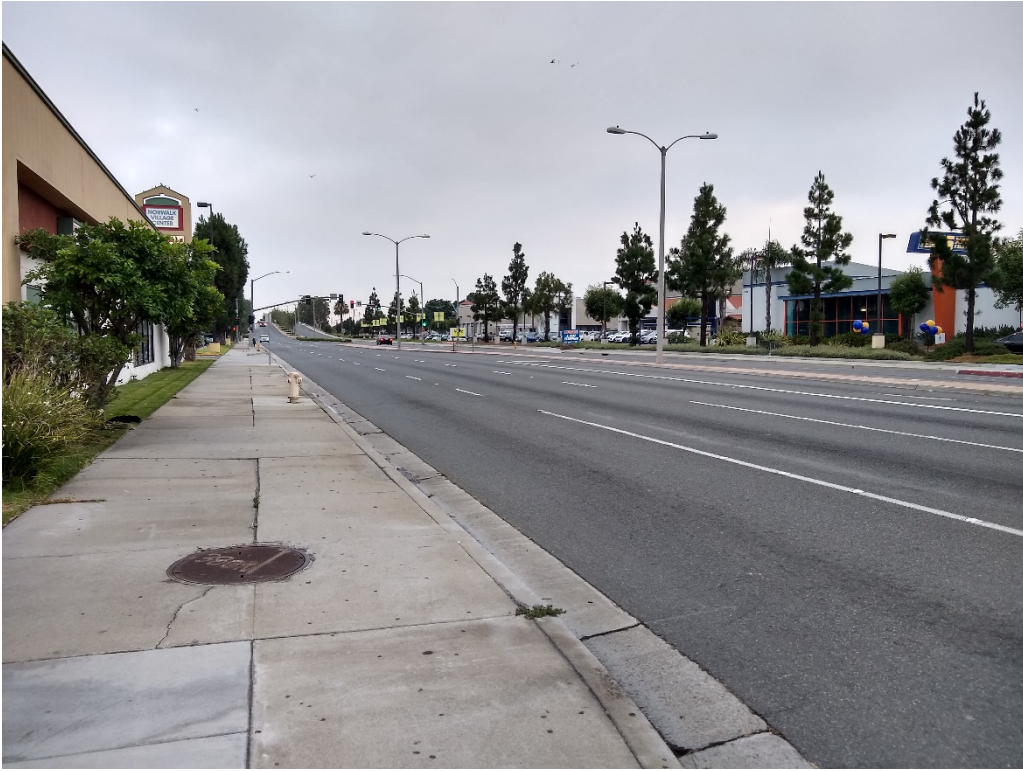
Photograph 3 – Firestone Boulevard near the I-605 northbound onramp, facing southeast.
