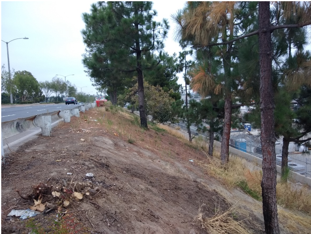
Photograph 6 – Firestone Boulevard, facing southeast.
