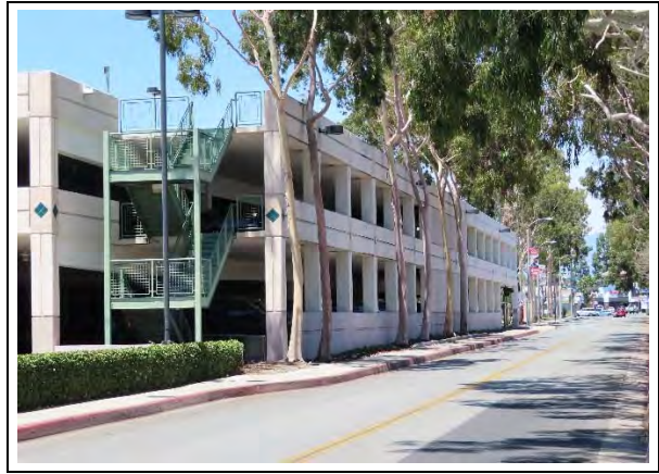
Parking structure, east façade, view northwest (ARG, 2022)
