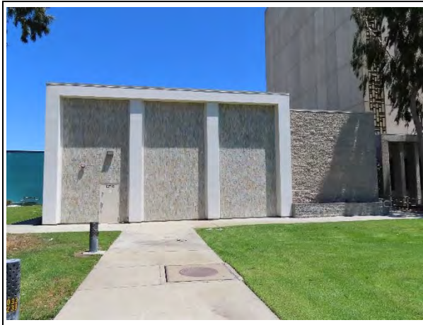
County accessory building, west façade, view east (ARG, 2022)
