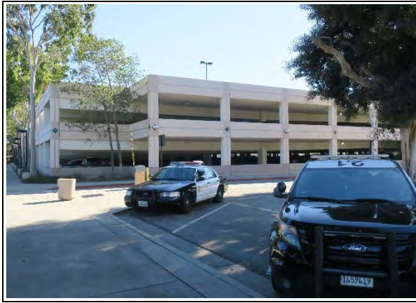
Parking structure, west façade, view southeast (ARG, 2022)
