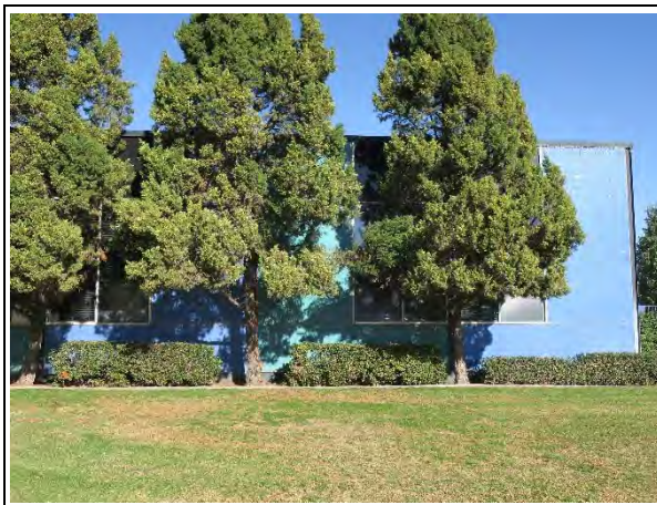
South façade, view north (ARG, 2022)
