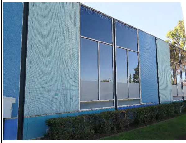
North façade, detail of wall tiles and aluminum windows (ARG, 2022)
