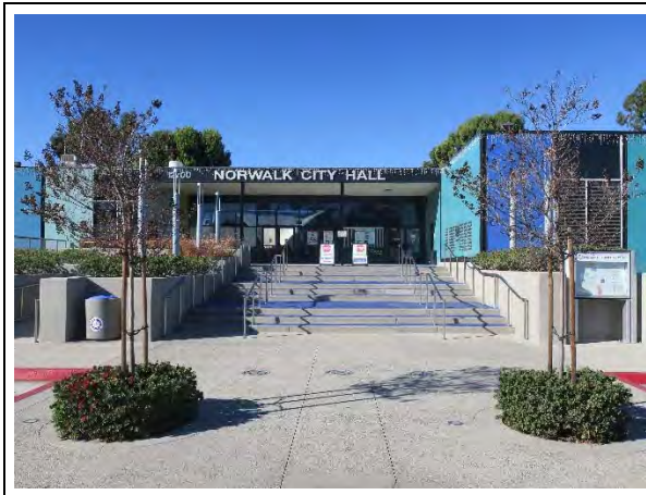
Rear (east) façade, view west (ARG, 2022)
