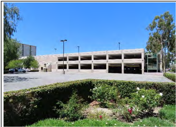
Parking structure, south façade, view northwest (ARG, 2022)
