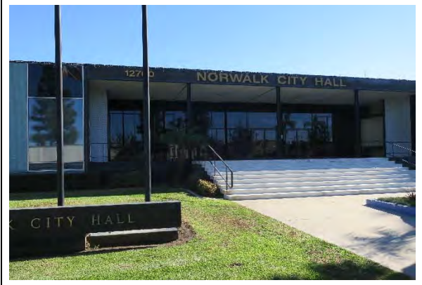
Primary (west) façade, view southeast (ARG, 2022)
