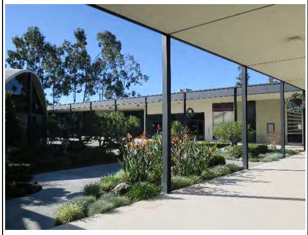
Building viewed from courtyard, view northwest (ARG, 2022)
