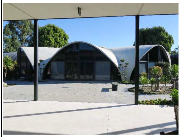
Circular volume at center of courtyard, view northeast. Note ribbed parabolic roof (ARG, 2022)
