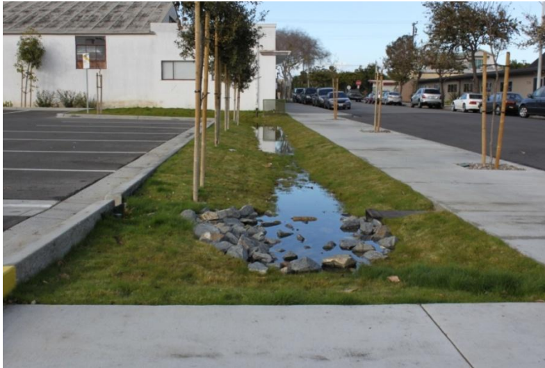
Figure 8: Vegetated swale ( Signal Hill, CA ).
