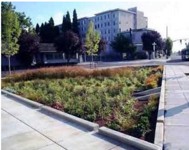
Figure 3: Rain garden ( Model for Living Streets Design Manual, 2011 ).
