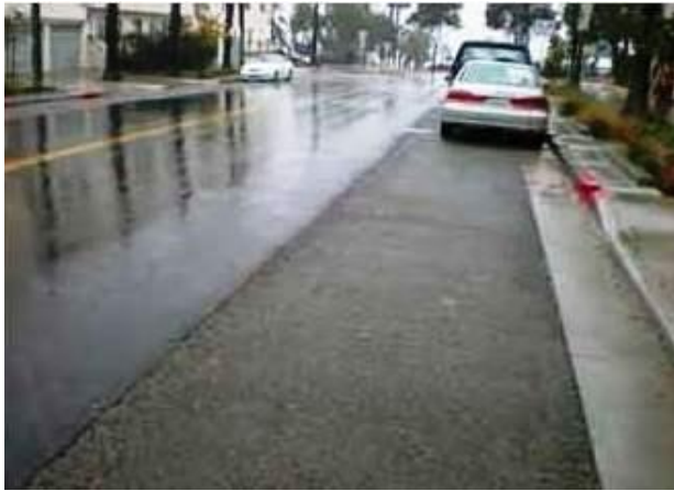
Figure 4: Permeable pavement during a storm event ( Model for Living Streets Design Manual, 2011 ).
